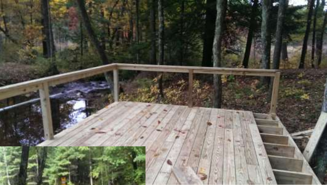
Construction of Handicap Accessible Viewing Station
