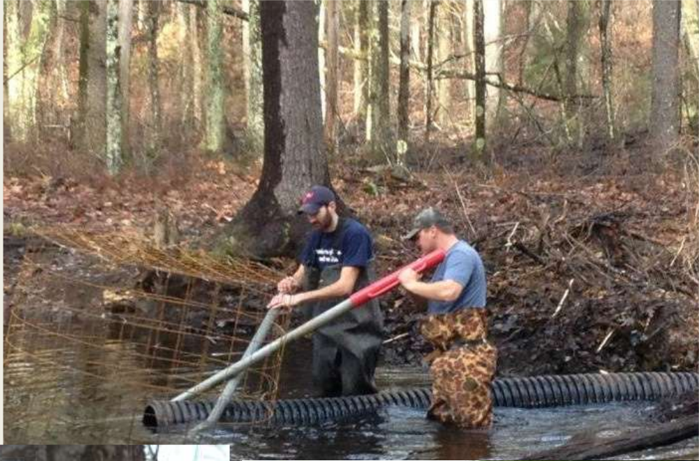
Construction of Beaver Control Devices
